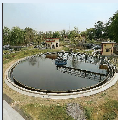
Treatment Plant, Allahabad
